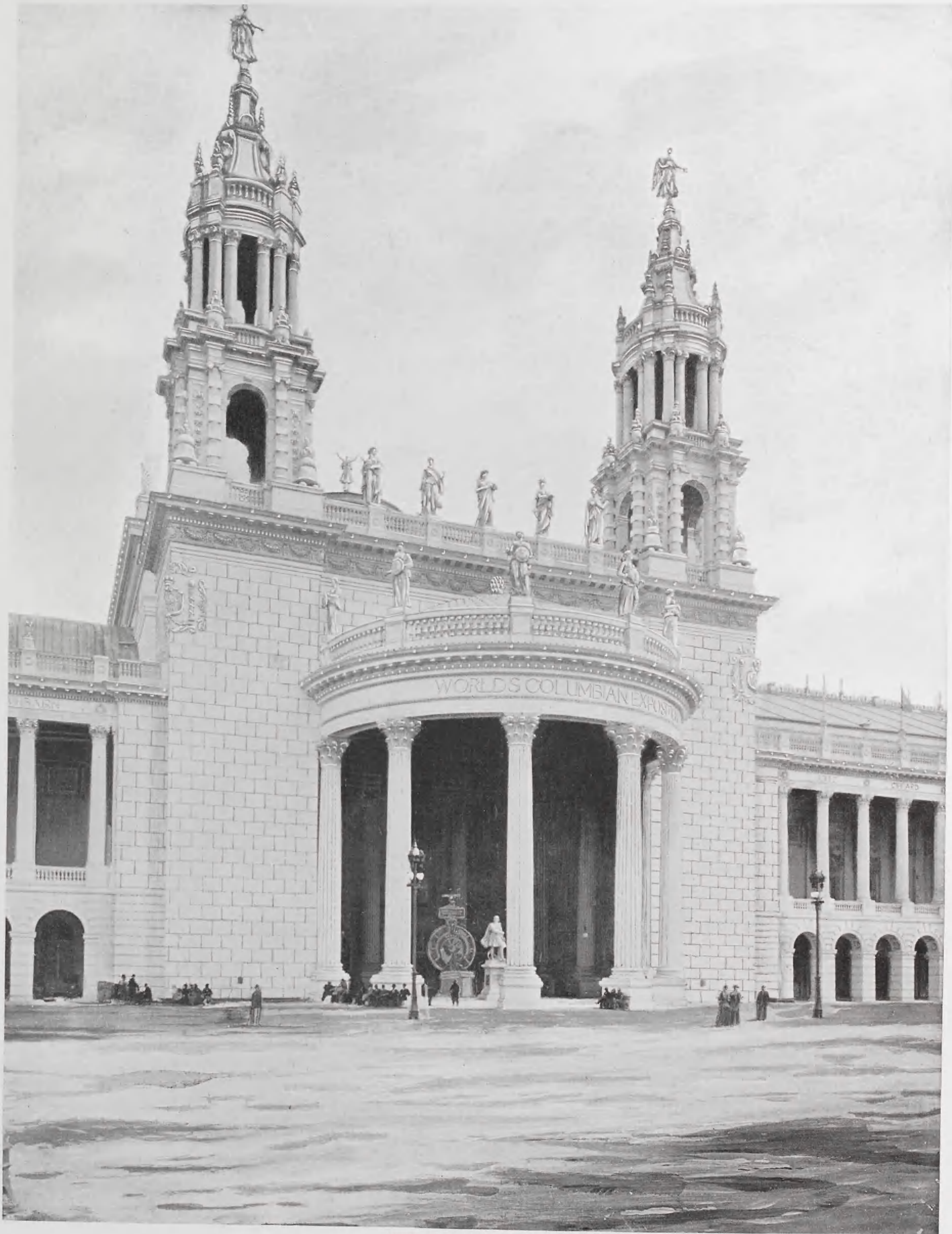
ENTRANCE MACHINERY BUILDING
